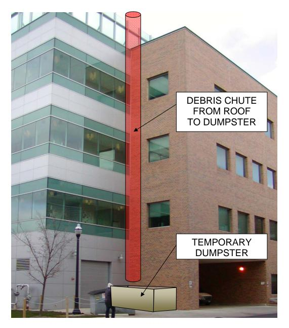
On or around December 14th and continuing throughout the Holiday break, FOD will have a dumpster and a debris chute positioned as shown. Contractors will be working on the roof to remove damaged insulation that was blown off of a large area of external ductwork during the windstorm of September 2008.
